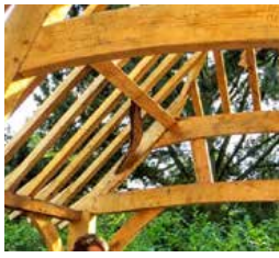
Woodland Barn built in 2013, before the shingles were added
